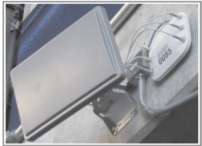
Fig. 4. Cisco 3502P AP with grayling antenna.
