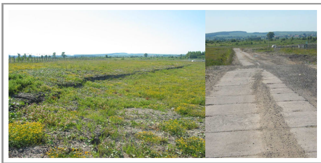
Fig. 6. Surface and local road degradation on the Jaroszów landslide.
